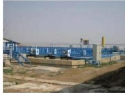
**4. Sedimentation** - The water next enters the sedimentation basin. The floc settles to the bottom of the basin having the dimensions of 48x16x7.5 m to remove the impurities from the water. The water then proceeds to the filtration stage.
