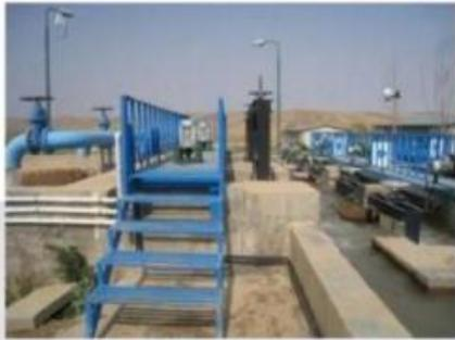
**2. Rapid Mixing** - The water arrives at the treatment plant into two rapid mixing pools each with the capacity of 3.375 m<sup>3</sup>, where coagulants ( that cause fine particles to clump together, forming "floc") are added. This mixing disperses the coagulants throughout the water and starts the coagulation process
