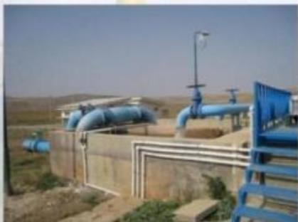
**3. Slow Mixing** - The water then passes through four flocculation pools in three steps each with the capacity of 33.075 m<sup>3</sup>, where it is gently mixed. This causes the particles to come together and form larger floc.
