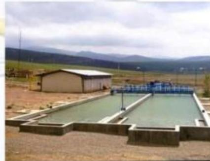
**5. Filtration** -From the sediment basin, the water flows through 12 units of pressure filters. As the water passes through the filter, impurities stick to the filter material
